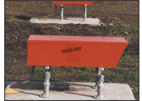
Four legs equipped with frangible floor flanges provide extra stability.
